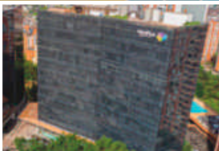
BIO 26 HOTEL & BUSINESS CENTER - TORRE 3, MEDELLÍN ARQUITECTO: OPUS CONSTRUCTOR: OBRASDÉ
